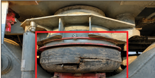
Coiled Spring Cracked/Broken/Sifted Detected
